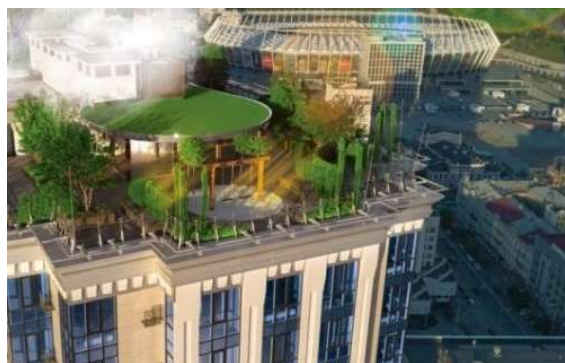
Figure 3 – Green roof of the Royal Tower
