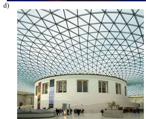
Figure 1 – Examples of the diagrid structural systems:
