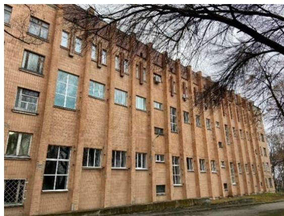
Figure 2 – Side facade of the educational building
