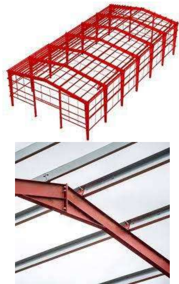
Figure 1 – General view of a steel framework and purlins
