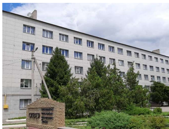
Figure 1 – An example of successful facade thermal modernization
