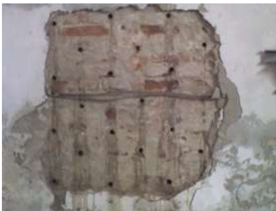
Figure 3 – Perforated wall grid
