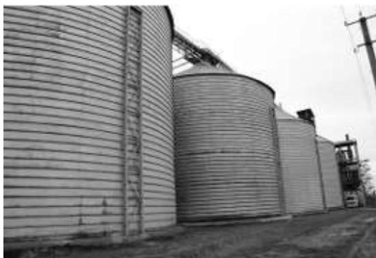
Figure 6 – Spiral-fold silos (elevator in village Emylivka, Kirovohrad region, 1971)
