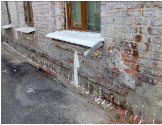
Figure 2 – General view of the experimental external wall
