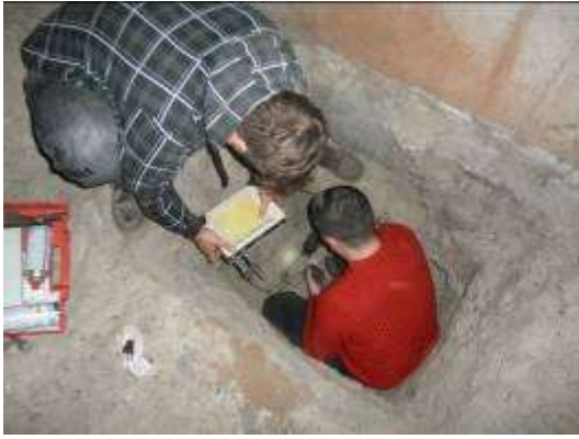
Figure 7 – Performing pile length control work
