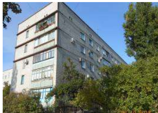
Figure 2 – View of the left side block section in the axes A-B and on the axis A
