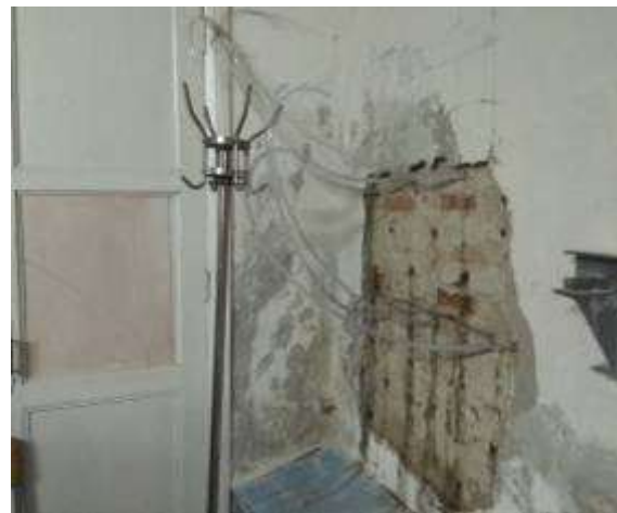
Figure 4 – The first type of experimental installation for injection waterproofing
