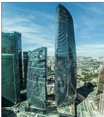
Figure 13 – Modern complex «Federation», Moscow, Russia
