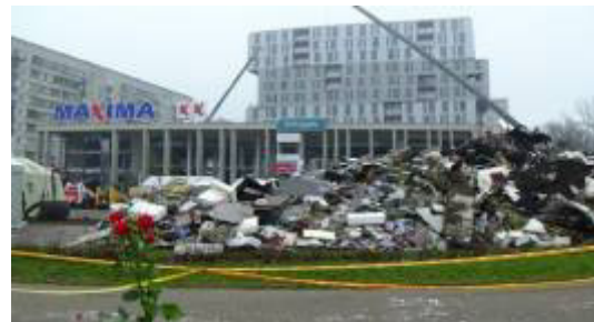
Figure 10 – The collapse of the Maxima Shopping Center in Riga, 2013
