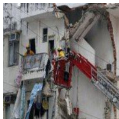
Figure 1 – Building collapse in Hong Kong, 2010
