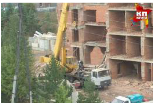
Figure 4 – The destruction building during construction, Ural, Russia, September 2016
