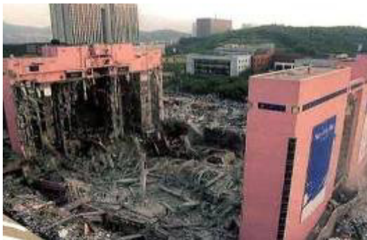
Figure 8 – Collapse of the Sampoong shopping center, Seoul, South Korea, 1995
