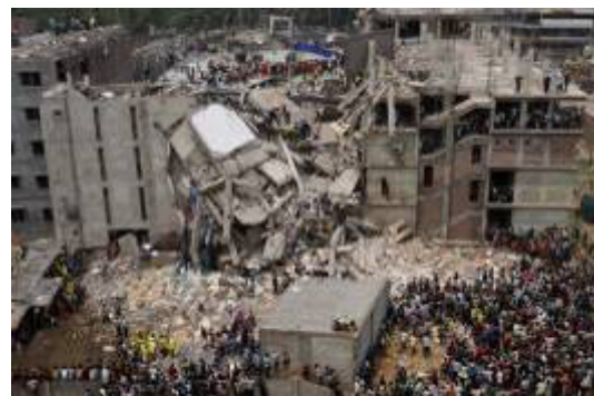
Figure 11 – Collapse of the complex in the city of Savar (Bangladesh), 2013
