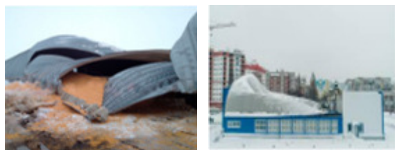
2017, The collapse of the granary (Ukraine)
