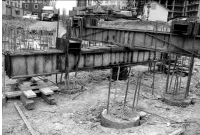
Figure 5 – Fragment of soils testing with bored piles
