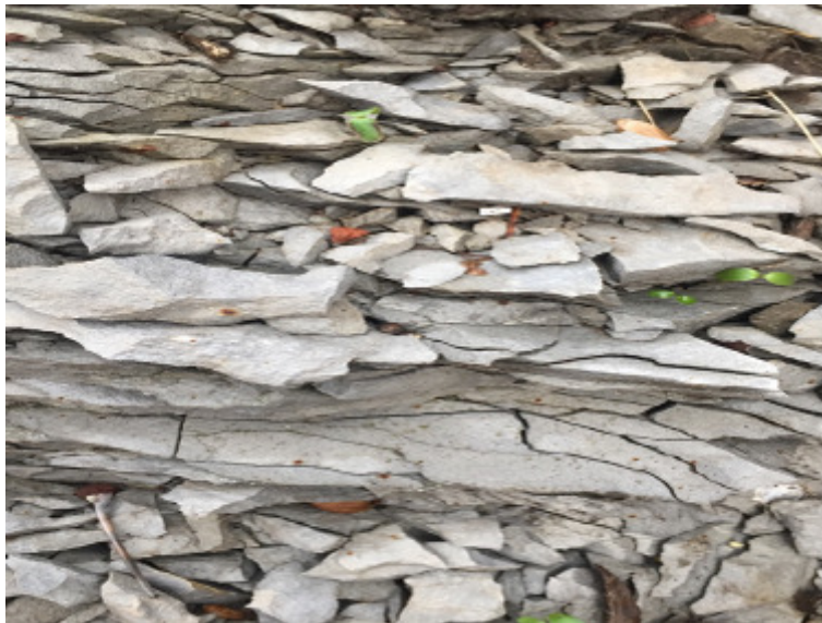
Figure 3 – Material bundle under weather conditions influence
