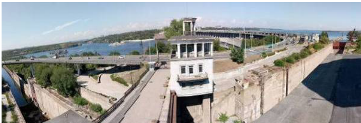
Figure 1 – General view of a three-chamber navigation lock in Zaporizhzhia city
