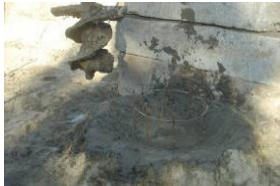
Figure 2 – Vibroreinforcing of soil-cement pile
