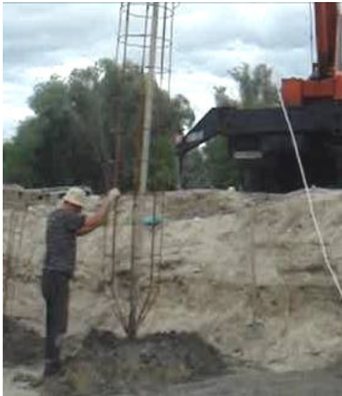
Figure 2 – Vibroreinforcing of soil-cement pile
