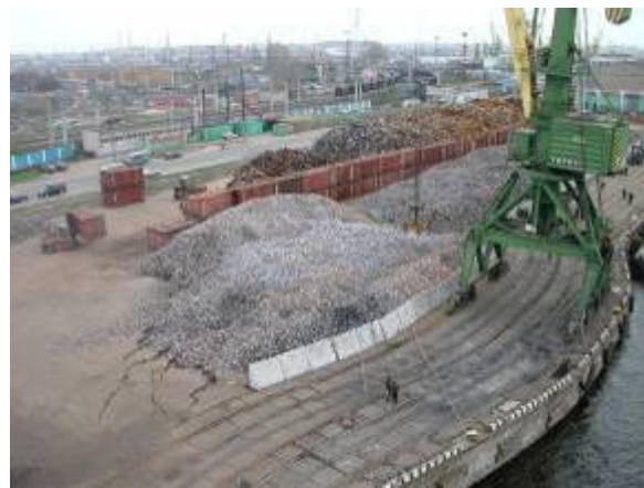
Figure 2 – Deformation of the berth due to overloading
