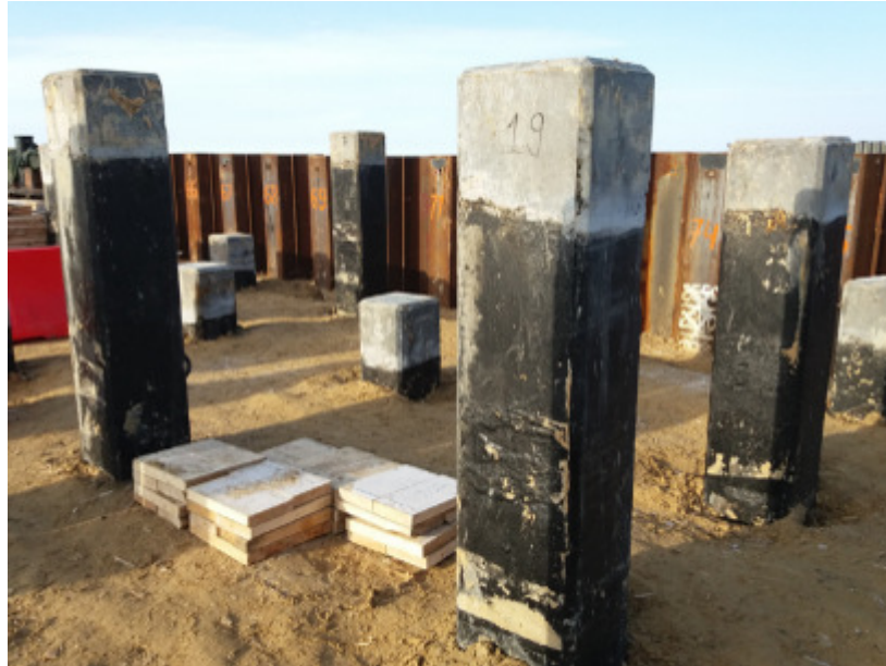
Figure 2 – Precast concrete pile on the site
