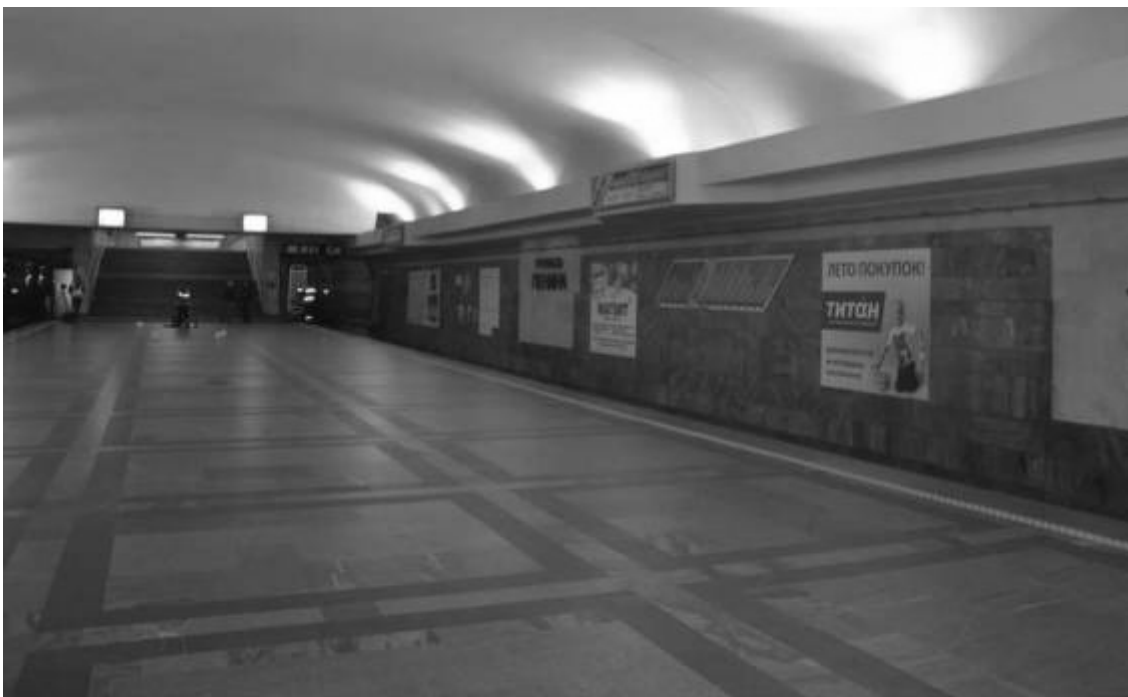
Figure 1 – General view of the platform site of the station before reconstruction
