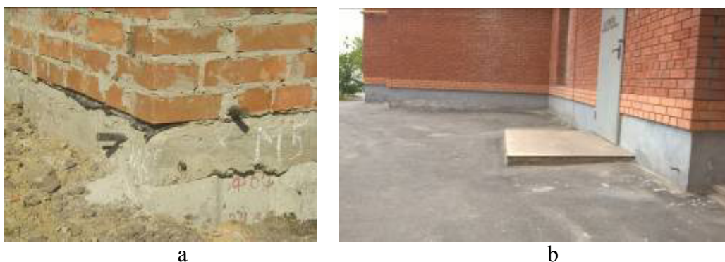
Figure 2 – Wall siege marks at the research object: a – at the time of their arrangement; b – at the time of leveling 01.10.2017
