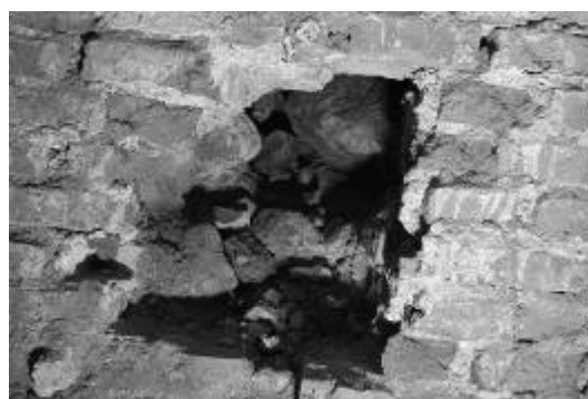
Figure 3 – Results of the structure opening to determine the technical state of foundations under the pillars
