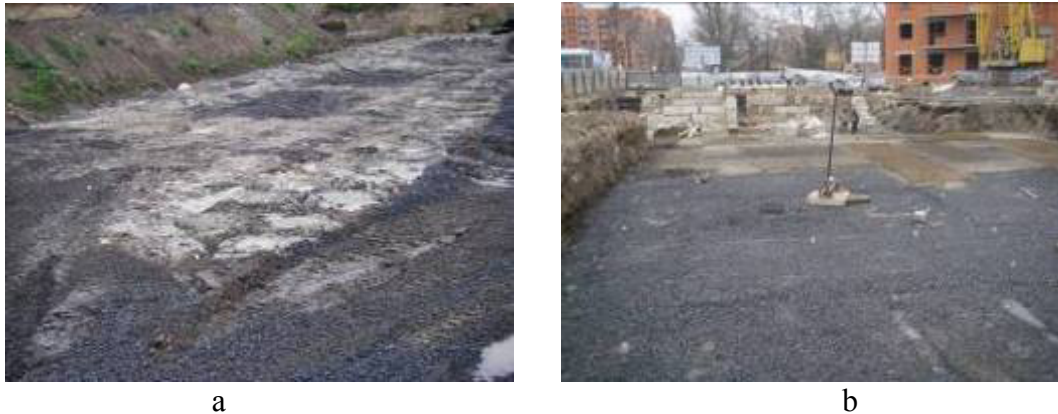
Figure 1 – The bottom of the foundation pit (sections IV and V) after reinforcing the SCE of the base (a), the gravel pillow, sprinkled on top of this base, and the strip monolithic foundations (b)
