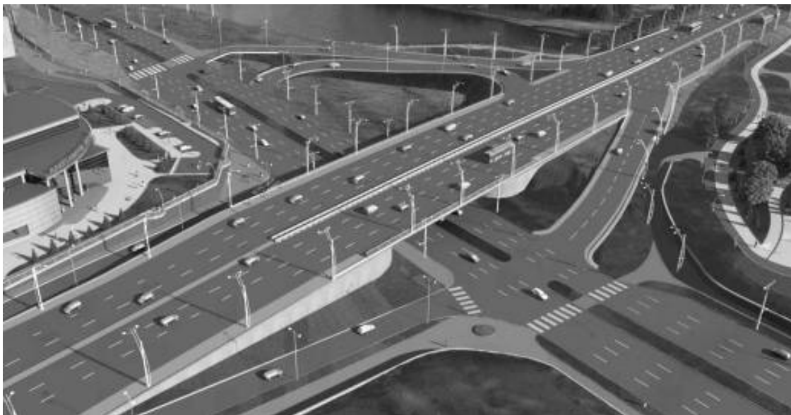
Figure 1 – General view of the projected transport interchange at the intersection Independence Avenue from the Filimonova Street
