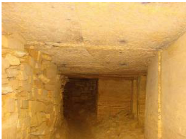
Figure 3 – General view of underground workings
