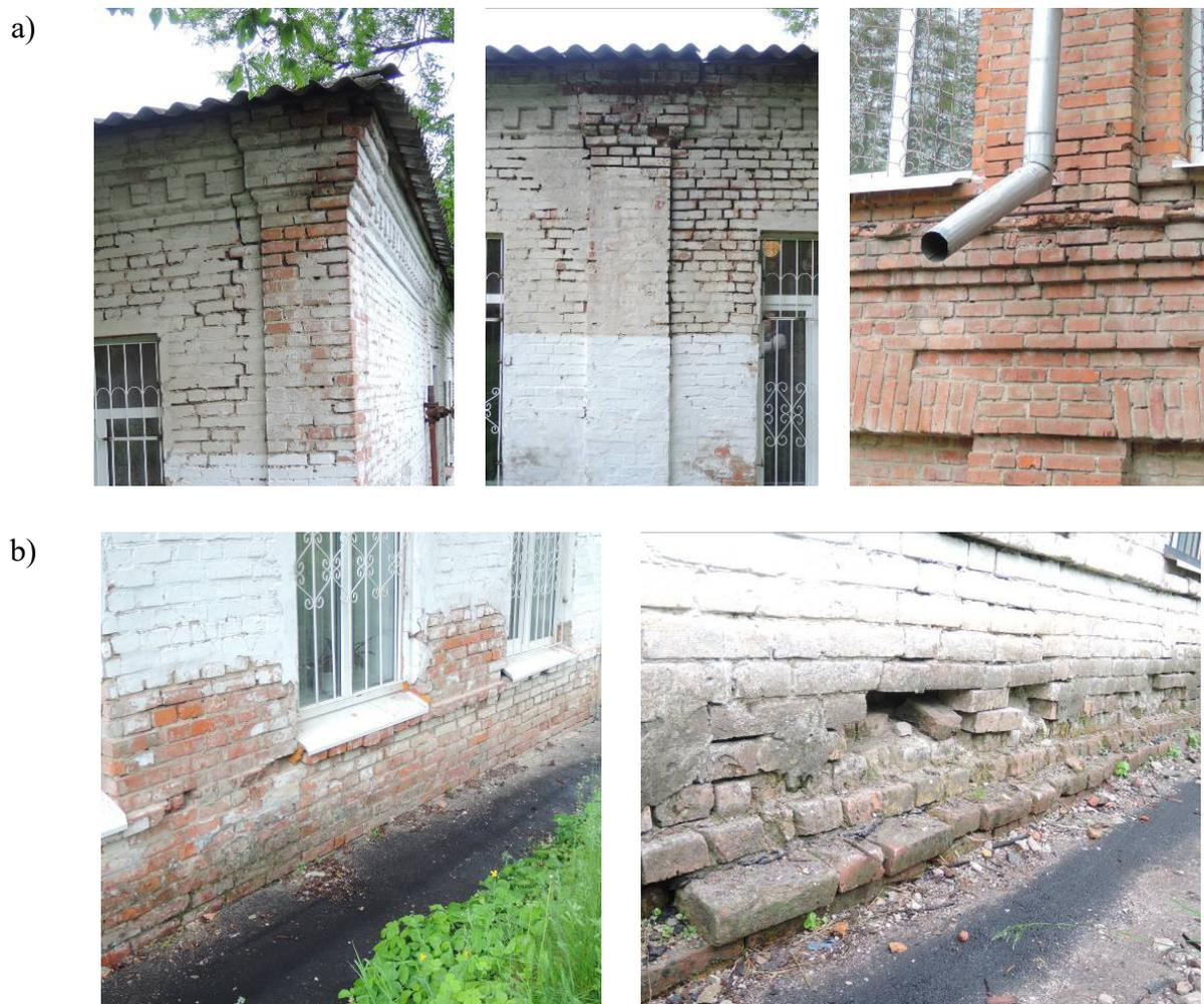
**Figure 2 – Atmospheric moisture effects to brickwork of buildings enclosing structures:**
