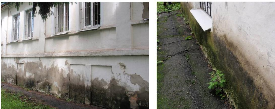
**Figure 4. – Soil moisture effect as a result of destruction or lack of horizontal waterproofing, in case of banked up building sidewalks level above the horizontal waterproofing level**
