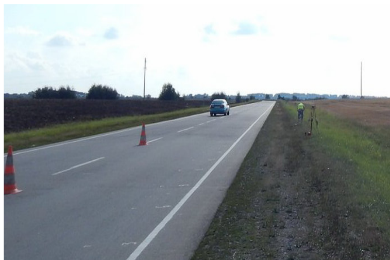
Figure 1 – General view of road section H-18 Ivano-Frankivsk – Buchach – Ternopil (km 63 + 098 – km 63 + 170)
