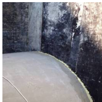
Figure 8 – Boards forming a pool over the cylindrical shell
