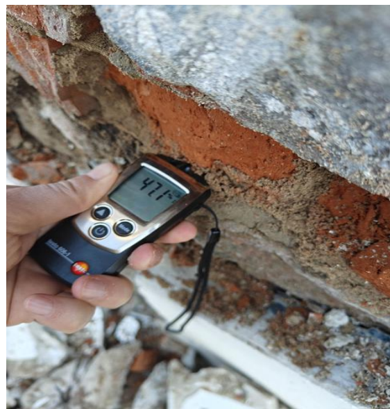
Figure 6 – Photos of moisture measurements of mortar and basement bricks
