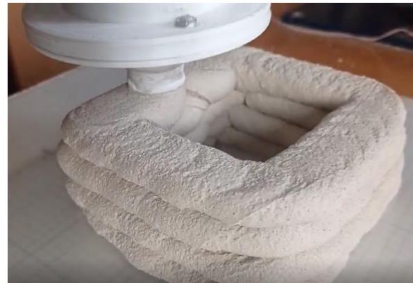
Figure 3 – The application of a layer of the concrete mixture onto the printing surface along a specified trajectory
