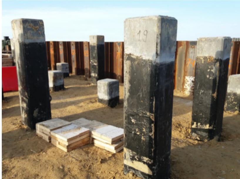
**Figure 2 – Precast concrete pile on the site**
