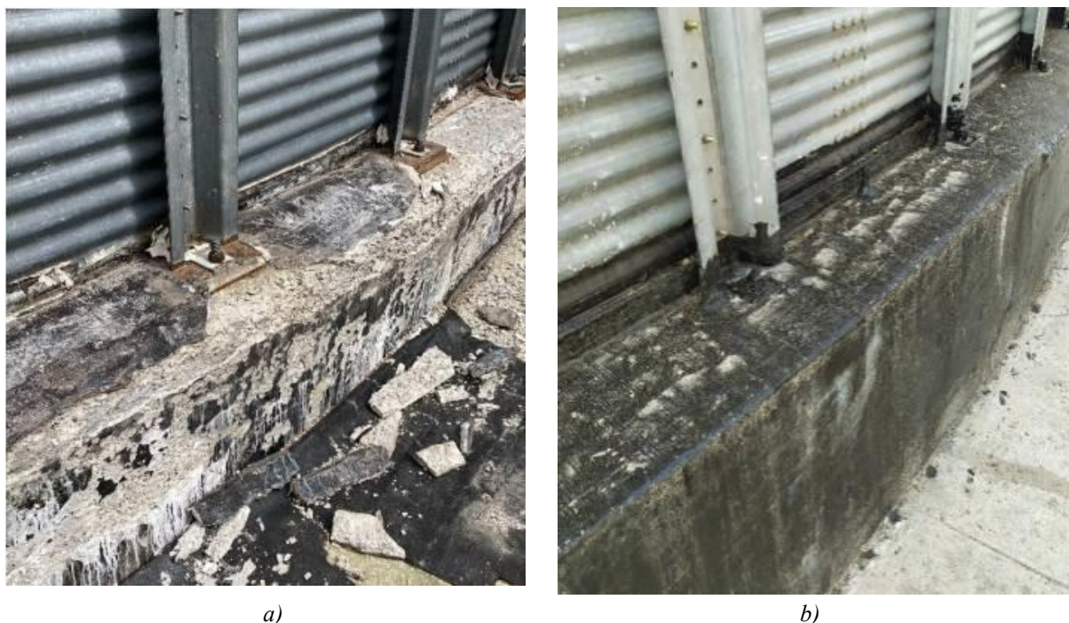
Figure 5 – Waterproofing of the above-ground part of the silo foundation: a) before repair; b) after repair
