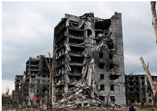
Figure 3 – The exterior of the destroyed building
