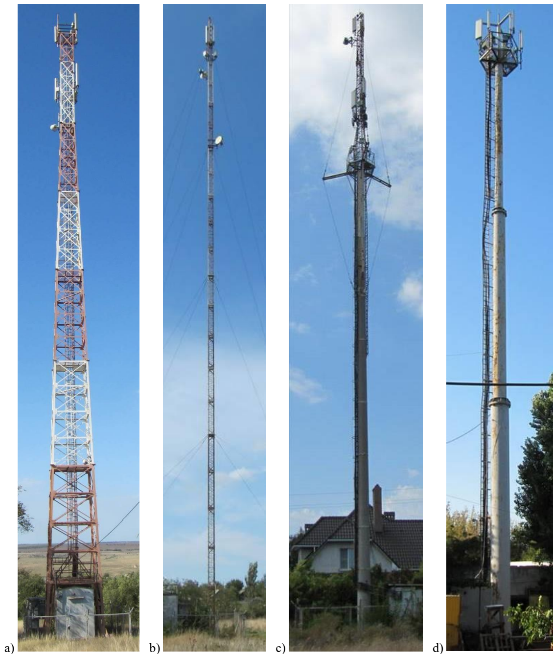
Figure 1 – General view of the tower (a), mast (b), combined support (c) and tubular tower (d)
