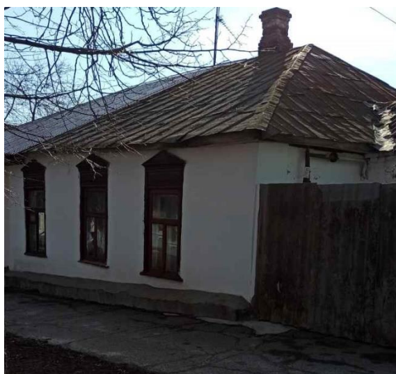
Figure 4 – Residential building with a "pryzba"
