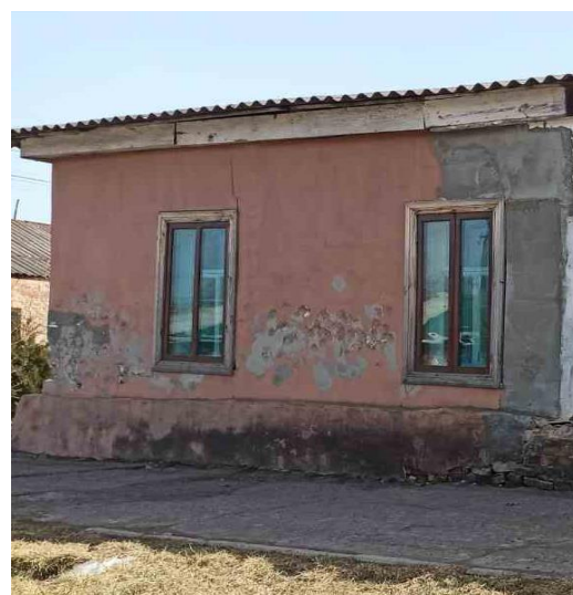
Figure 4 – Residential building with a "pryzba"
