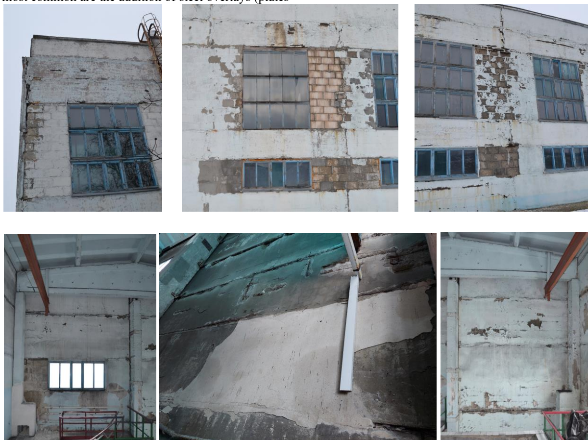
Figure 7 – Damage to wall panels
