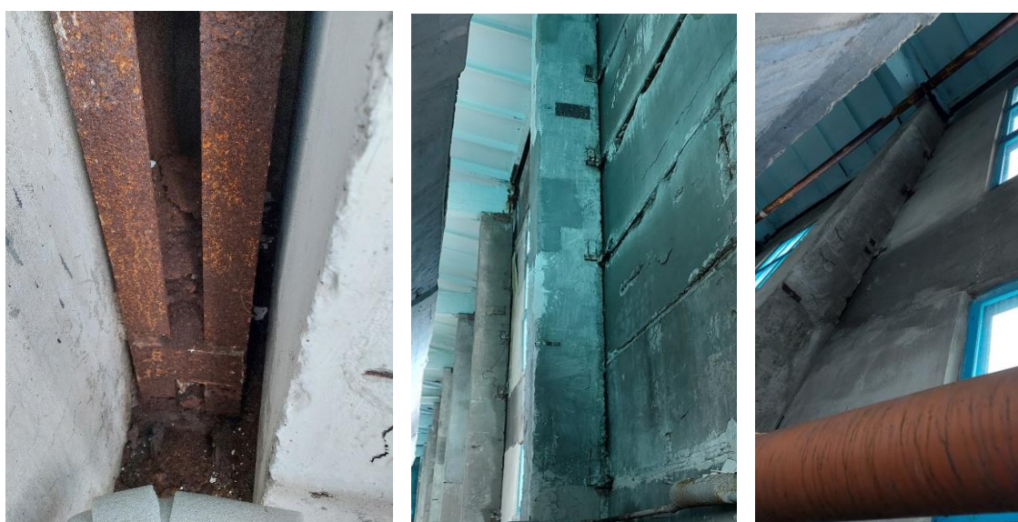
Figure 6 – Damage to half-timbered columns and metal embedded parts
