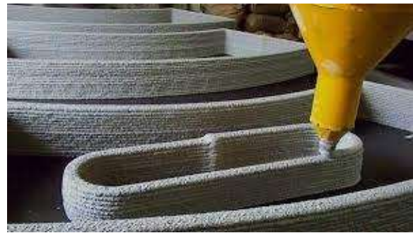
Figure 10 – Concrete extruding layer by layer
