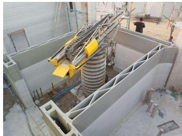
Figure 6 – Exhibition building by Apis Cor
