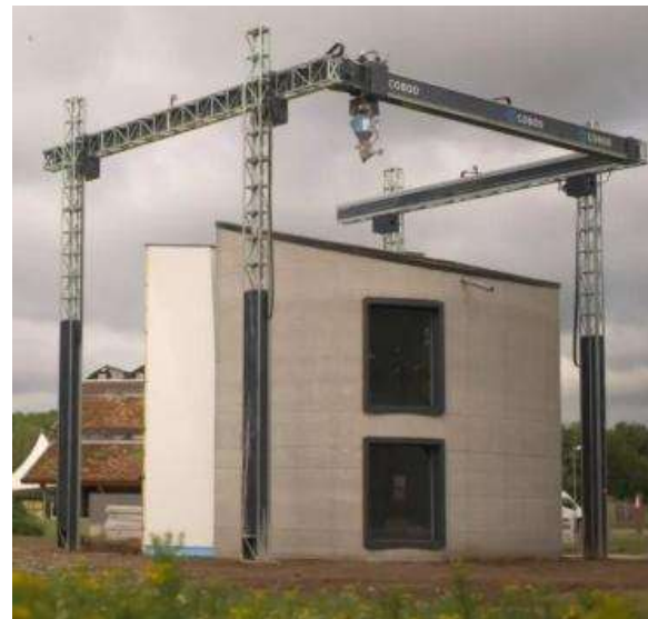
Figure 2 – Two-storey building printed by BOD2
