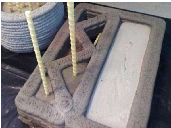
Figure 12 – Adding heat-insulating material or additional reinforcement
