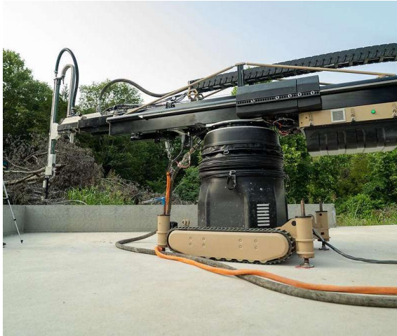
Figure 7 – 3D-printer by Apis Cor with tracked chassis
