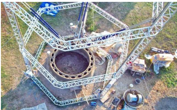
Figure 4 – 3D-printer Big Delta from WASP, Italy
