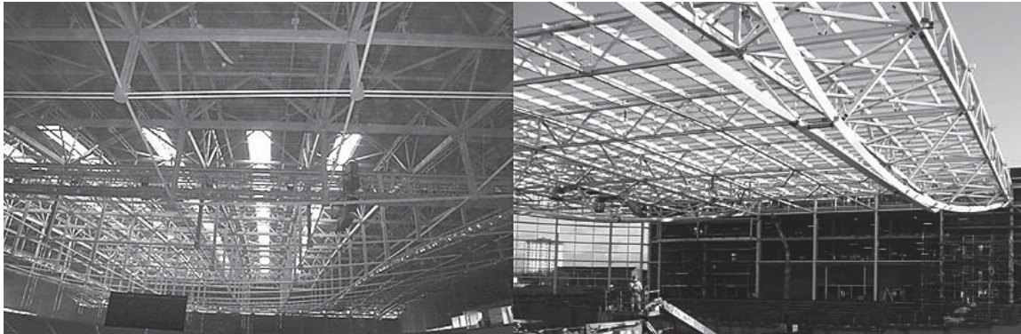
Figure 4 – Steel roof trusses of the National Indoor Stadium, Beijing
