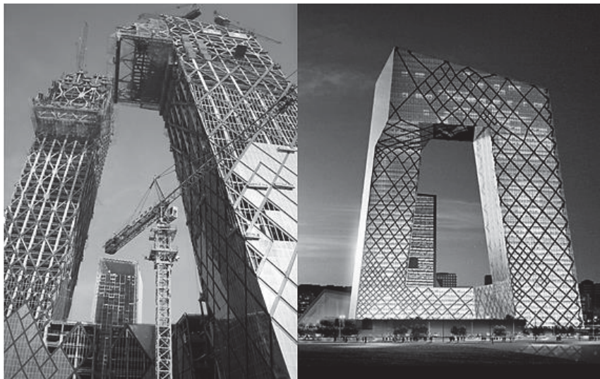
Figure 9 – View on CCTV Tower under construction (left) and the façade design of completed building (right)
