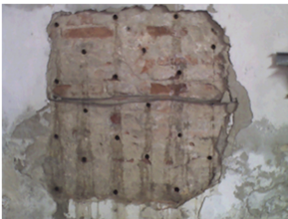
Figure 3 – Perforated wall grid
