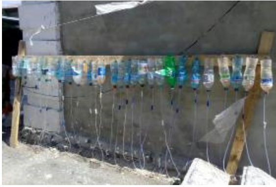
Figure 5 – The second type of experimental installation for injection waterproofing
