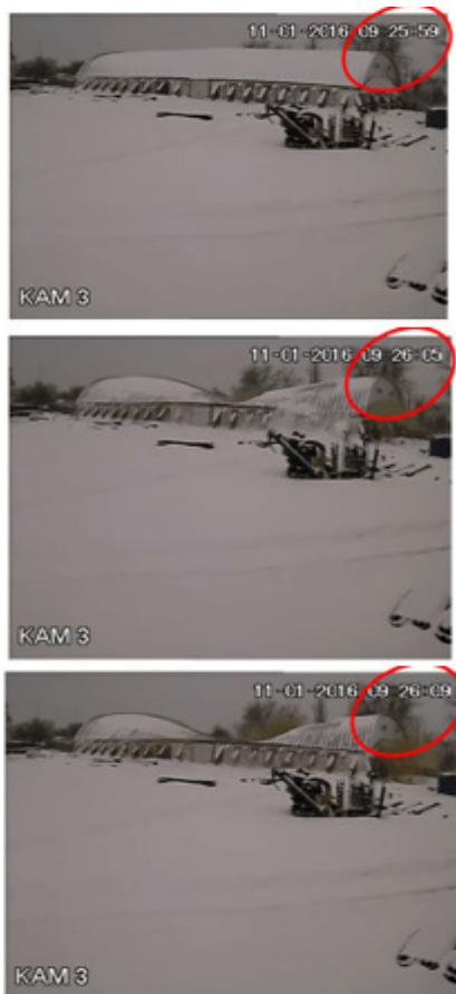
Figure 3 – A 60 meter long structure collapsed in less than 10 seconds
