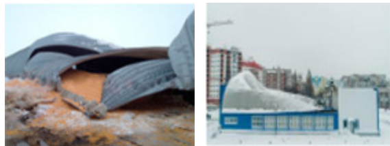
2017, The collapse of the granary (Ukraine)
