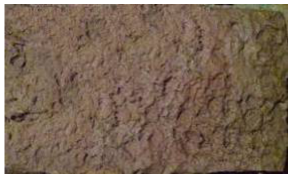
Figure 3 – The stand surface which was concreted by wet gunite method
