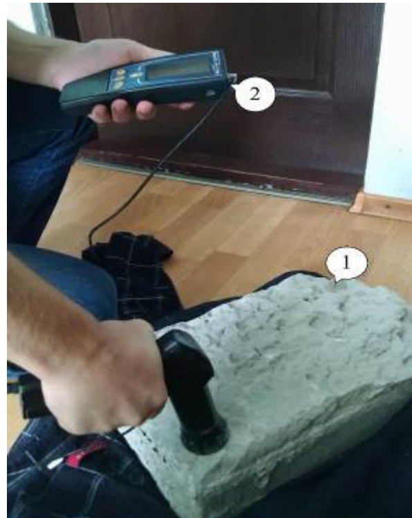
Figure 5 – The process of gunite concrete strength checking using the «Beton Pro Control» device:
