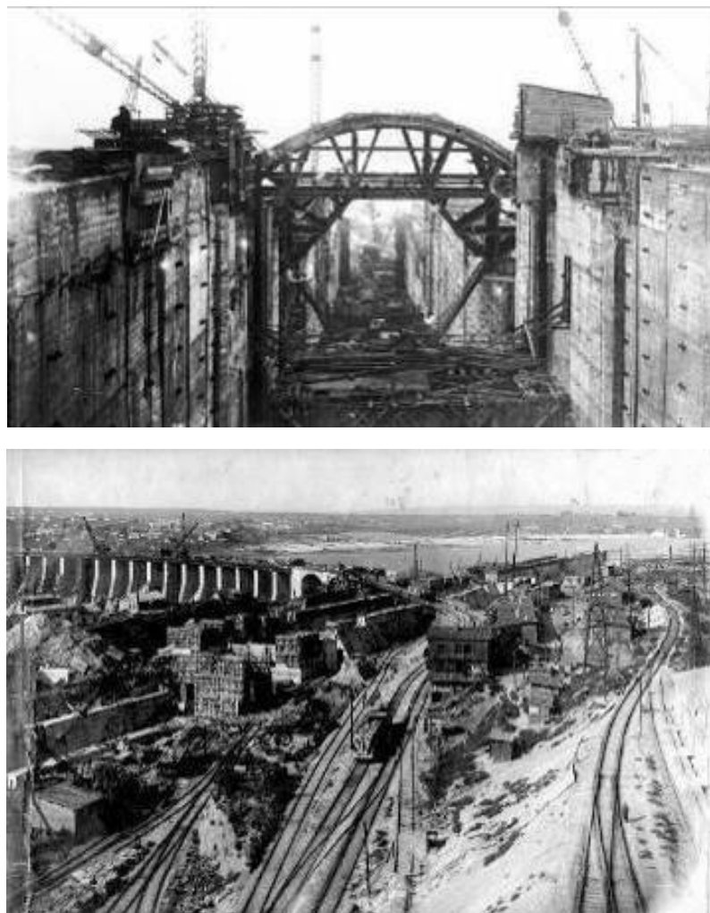
Figure 2 – General view of a three-chamber navigation lock in Zaporizhzhia city
