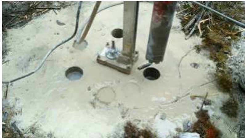
Figure 3 – General view of construction site with sampling area
