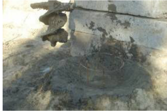
Figure 2 – Vibroreinforcing of soil-cement pile
