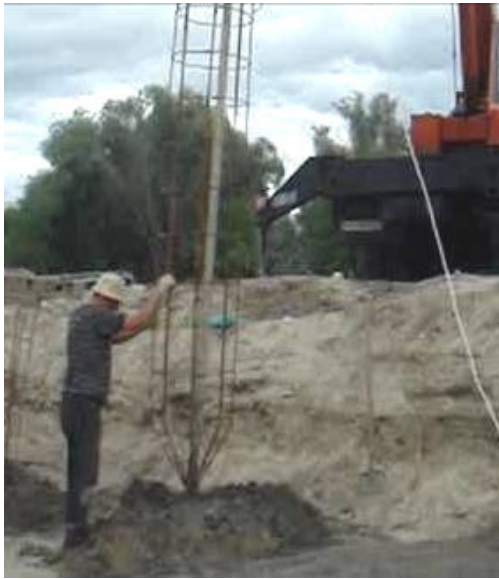
Figure 2 – Vibroreinforcing of soil-cement pile
