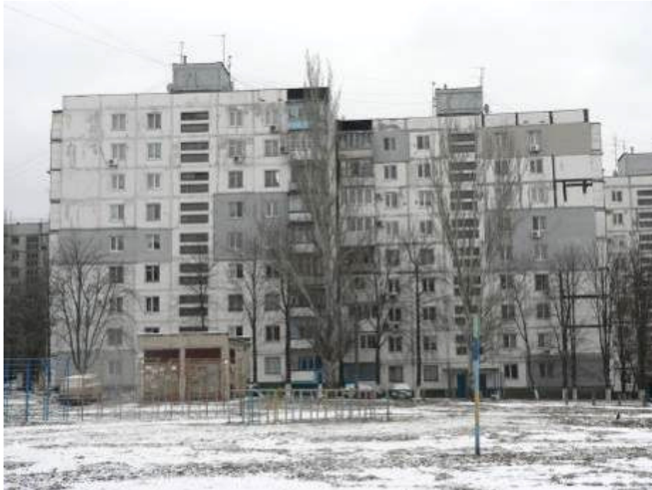
Figure 2 – General view of a residential building with collision of block-sections
